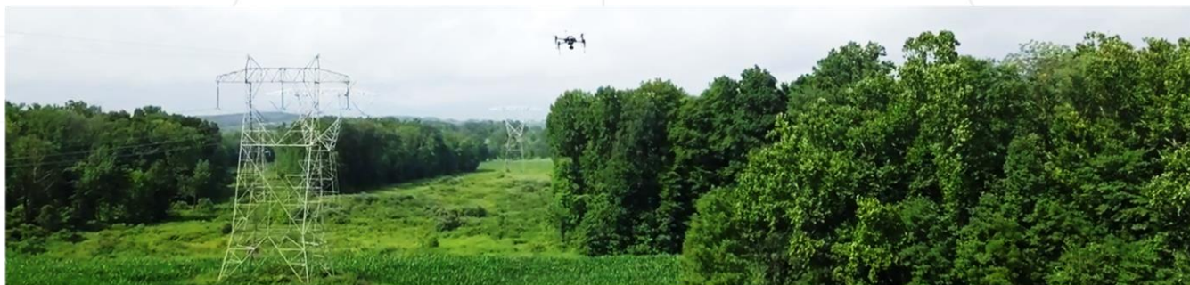
Photo courtesy of First Energy
